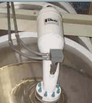
HRD suppression containers provide fast reaction time
