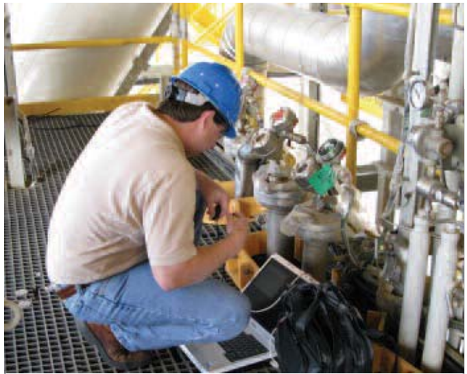
An Orion technician activates PACTware on a drilling rig.
